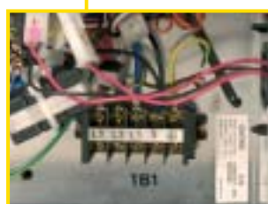
Outdoor unit power supply terminal block
