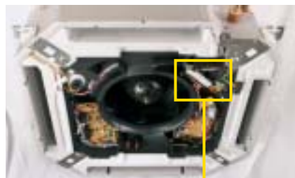
4-way cassette power supply connection
